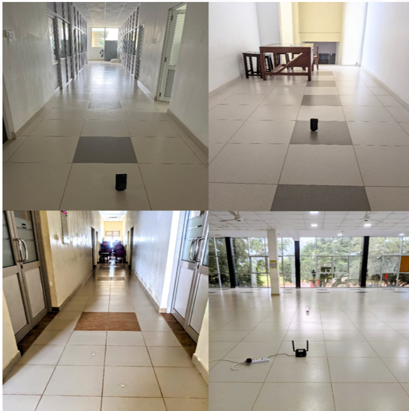
Figure 1. The study area is composed of different building elements and materials.
